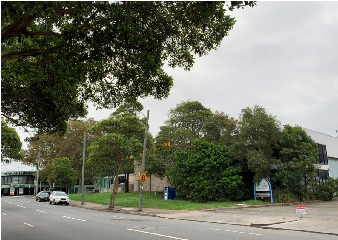
Figure 4: Looking south west towards 175-177 McEvoy Street (Petbarn)
