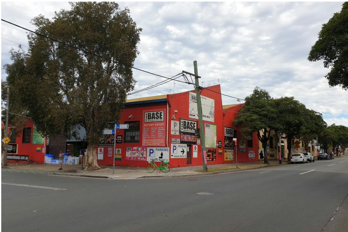
Figure 7: 132-138 McEvoy Street (Base Warehouse) located on the opposite side of the street. The site has approval for 4 storey commercial development.
