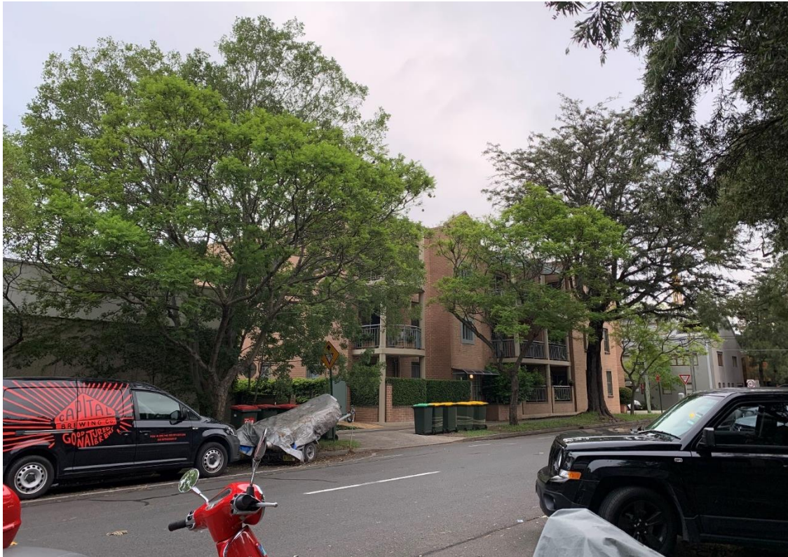
Figure 10: 118-136 Lawrence Street immediately to the west of the site
