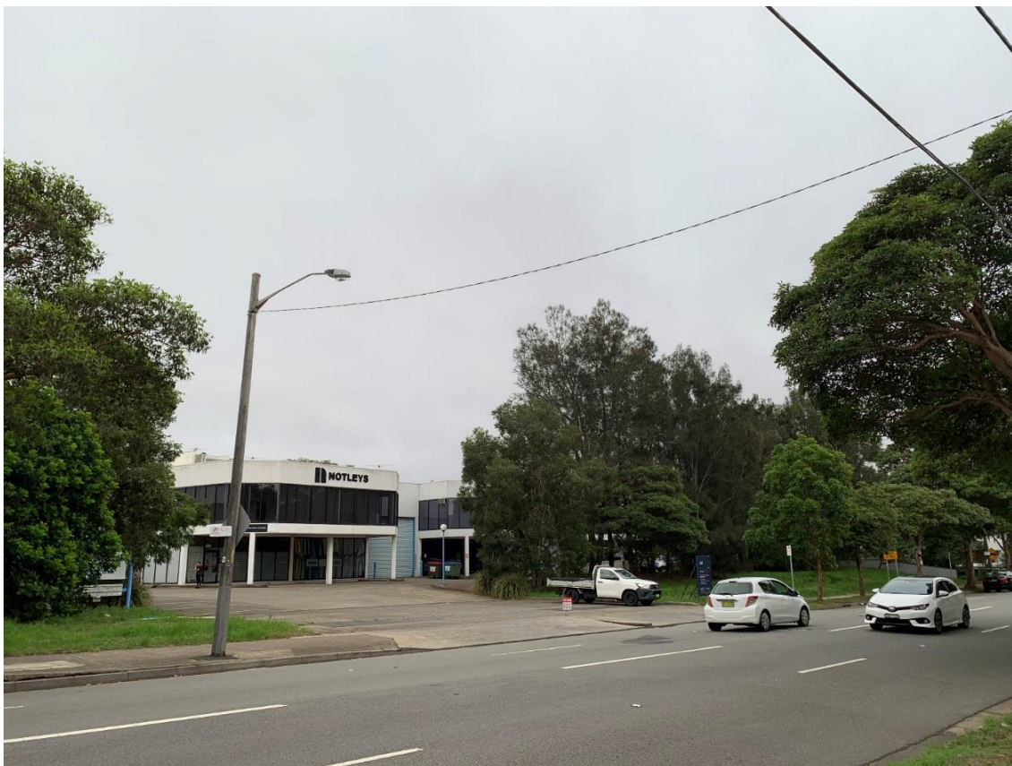
Figure 3: Site looking north from McEvoy Street
